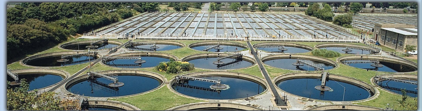
Water Reservoirs • Sewerage Ponds • Sewerage Channels Purification Ponds • Collection Dams • Water Storage
